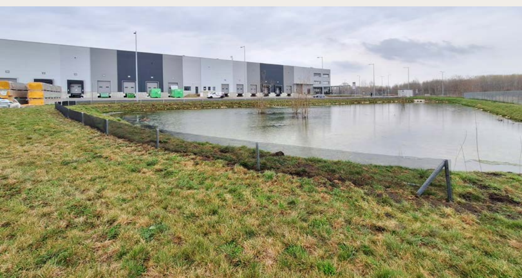
Existing pond at VGP Park Gyor Beta to be enhanced allowing several biodiversity improvements including artificial constructed brooding wall and ideal stepped lake bed and shoreline zonation
