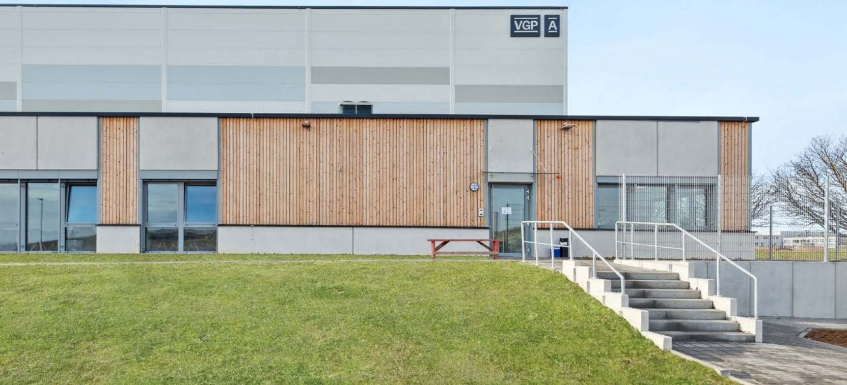
VGP Park Hochheim, Germany
