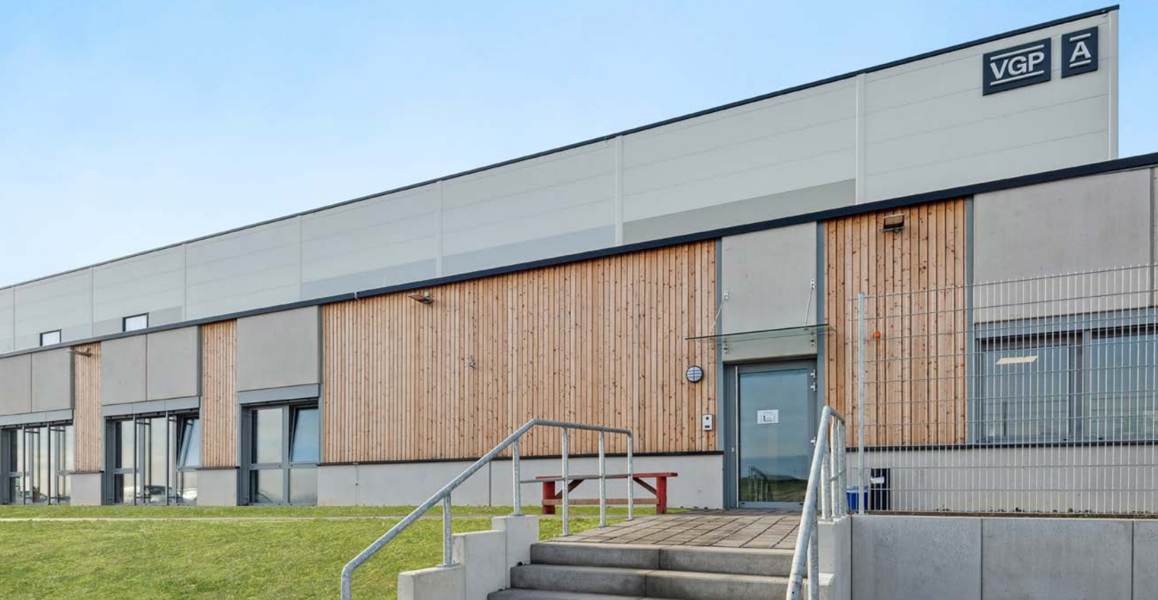
VGP Park Hochheim, Germany
