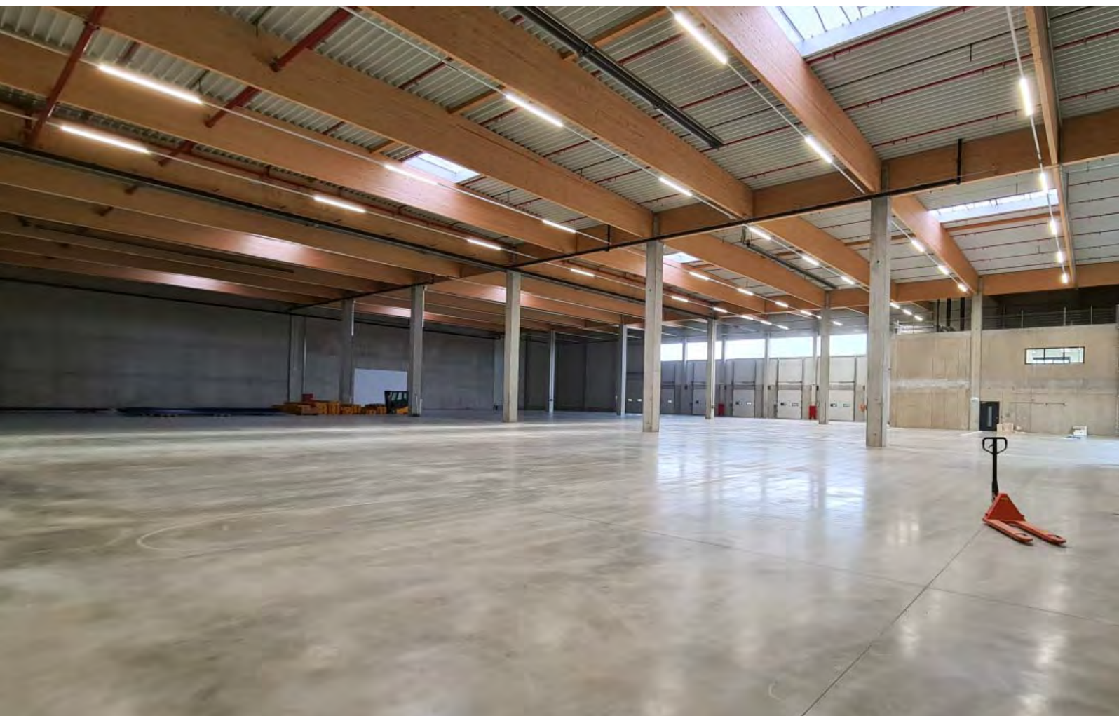
Wooden roof baring structure in VGP Park Graz
