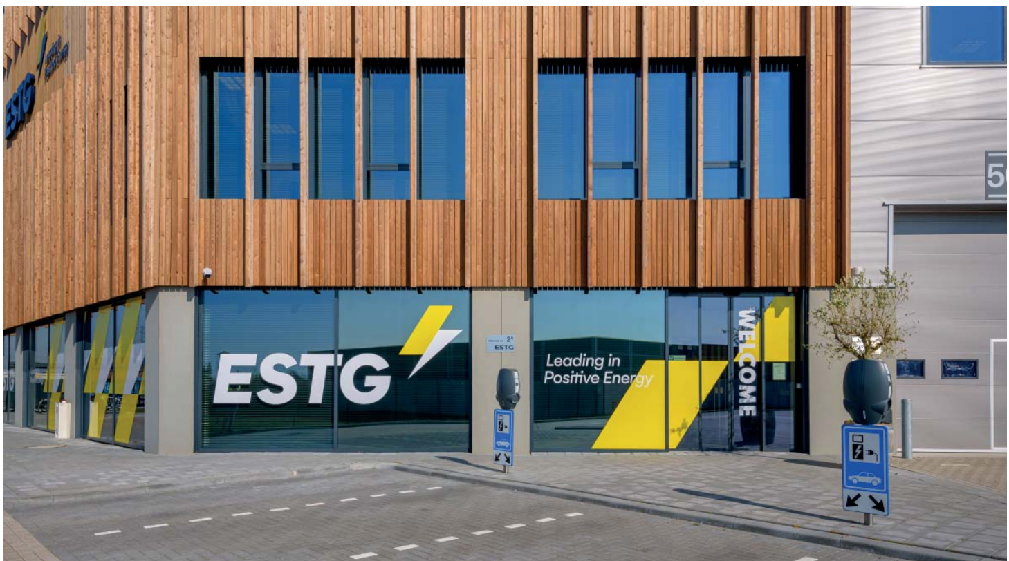
E-charging stations at VGP Park Nijmegen
