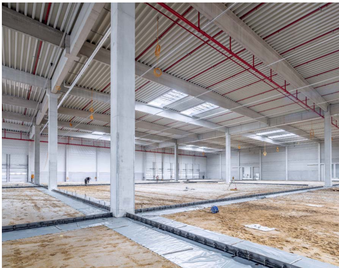
Works at VGP Park Soltau
