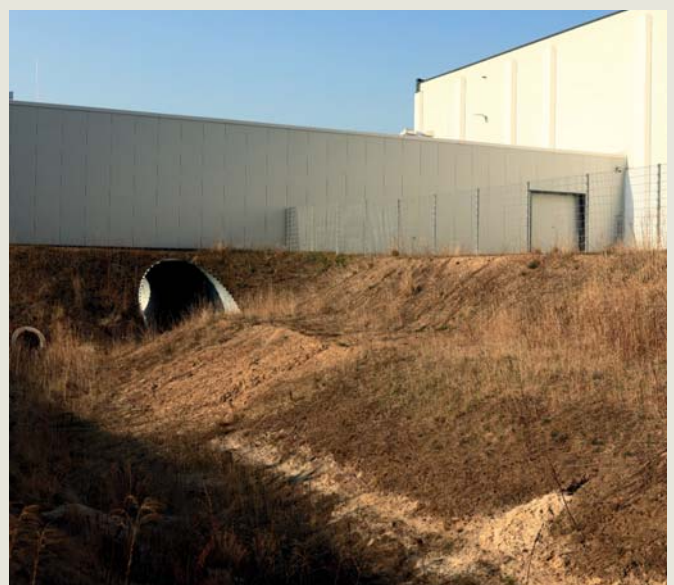
VGP Park Berlin – Water trenches to retain excess rainwater and ecoduct
