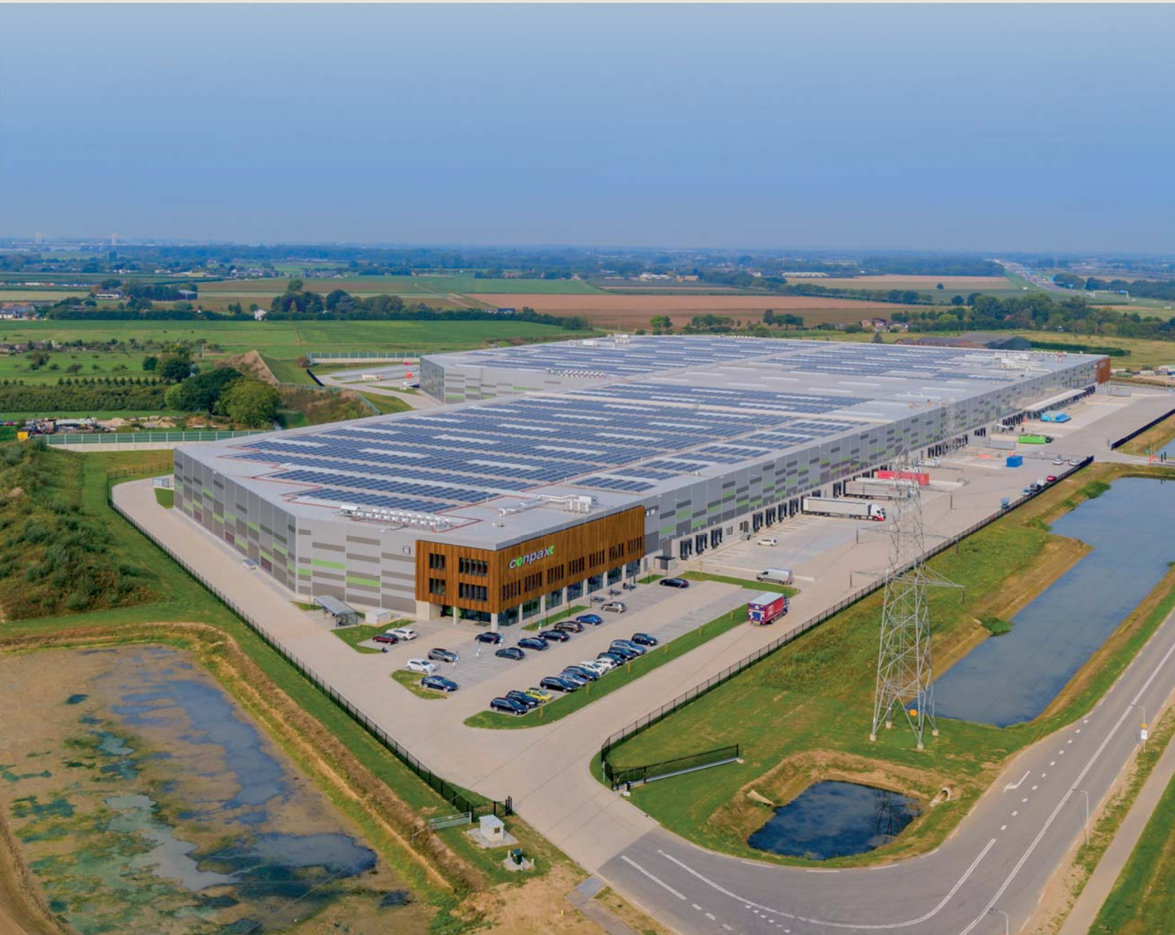
VGP Park Nijmegen with green walls and water retention bassin around the park.
