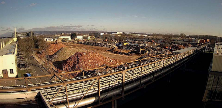
Demolition works at brownfield VGP Park Wiesloch-Walldorf with recyclable materials and soil being sorted and separated
