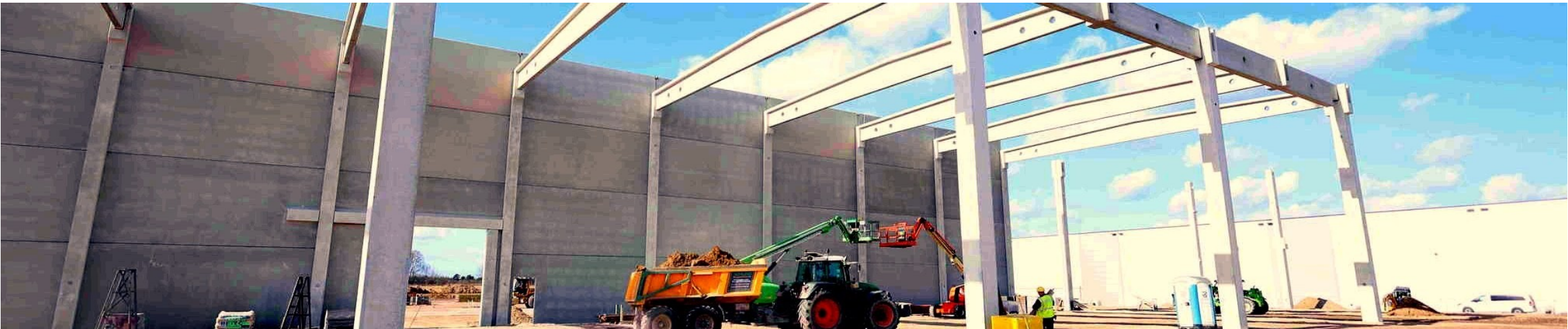
VGP Park under construction — precast frame, VGP as general contractor (photograph from the Capital Markets Day 2026 material).
