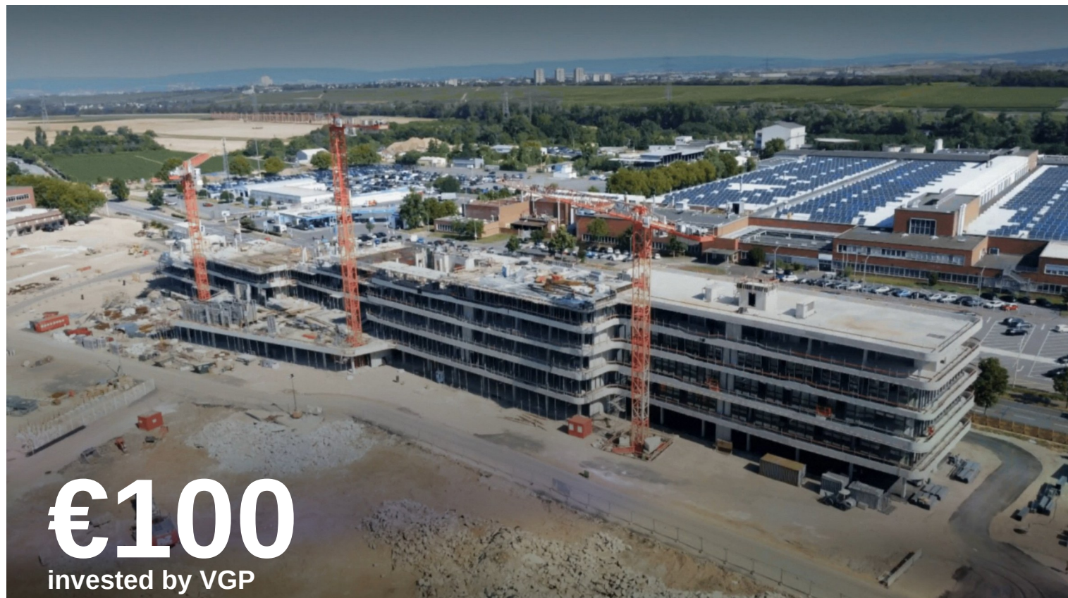
Construction phase — VGP Park Rüsselsheim, Green Campus Offices
