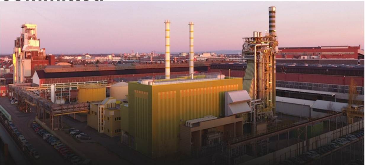
VGP Park Rüschelsheim — the on-site power infrastructure behind the “powered land” proposition (photograph)
