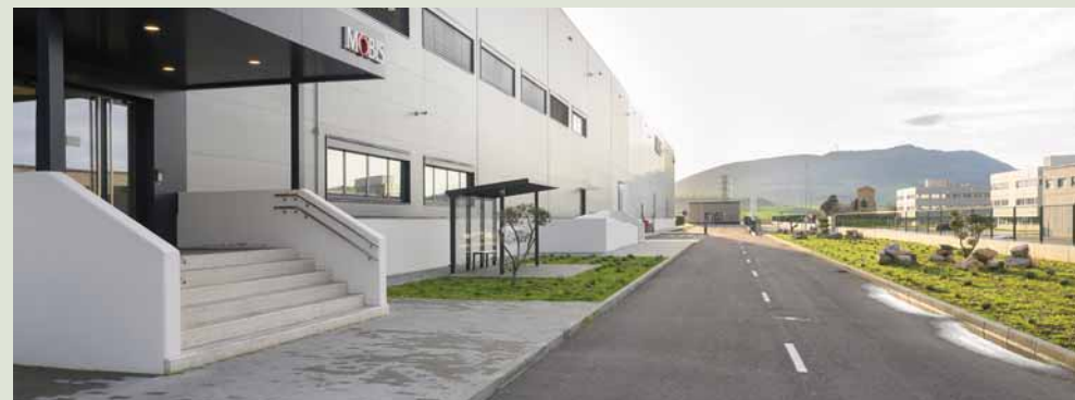
Perimeter green zone around the park
