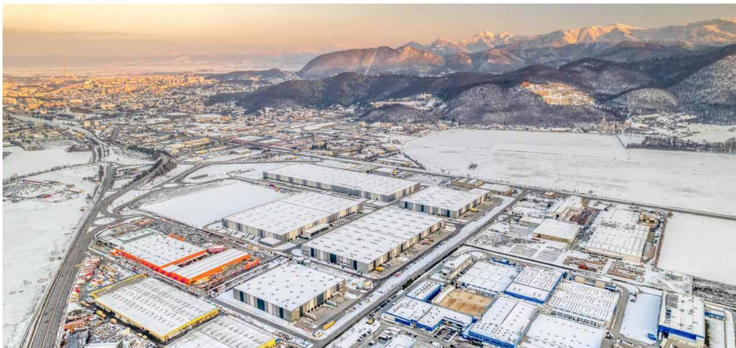
As winters grow more unpredictable, VGP Parks are designed to adapt – leveraging heat pumps, advanced insulation, and energy efficiency to reduce emissions while maintaining performance. (VGP Park Brasov, Romania)
