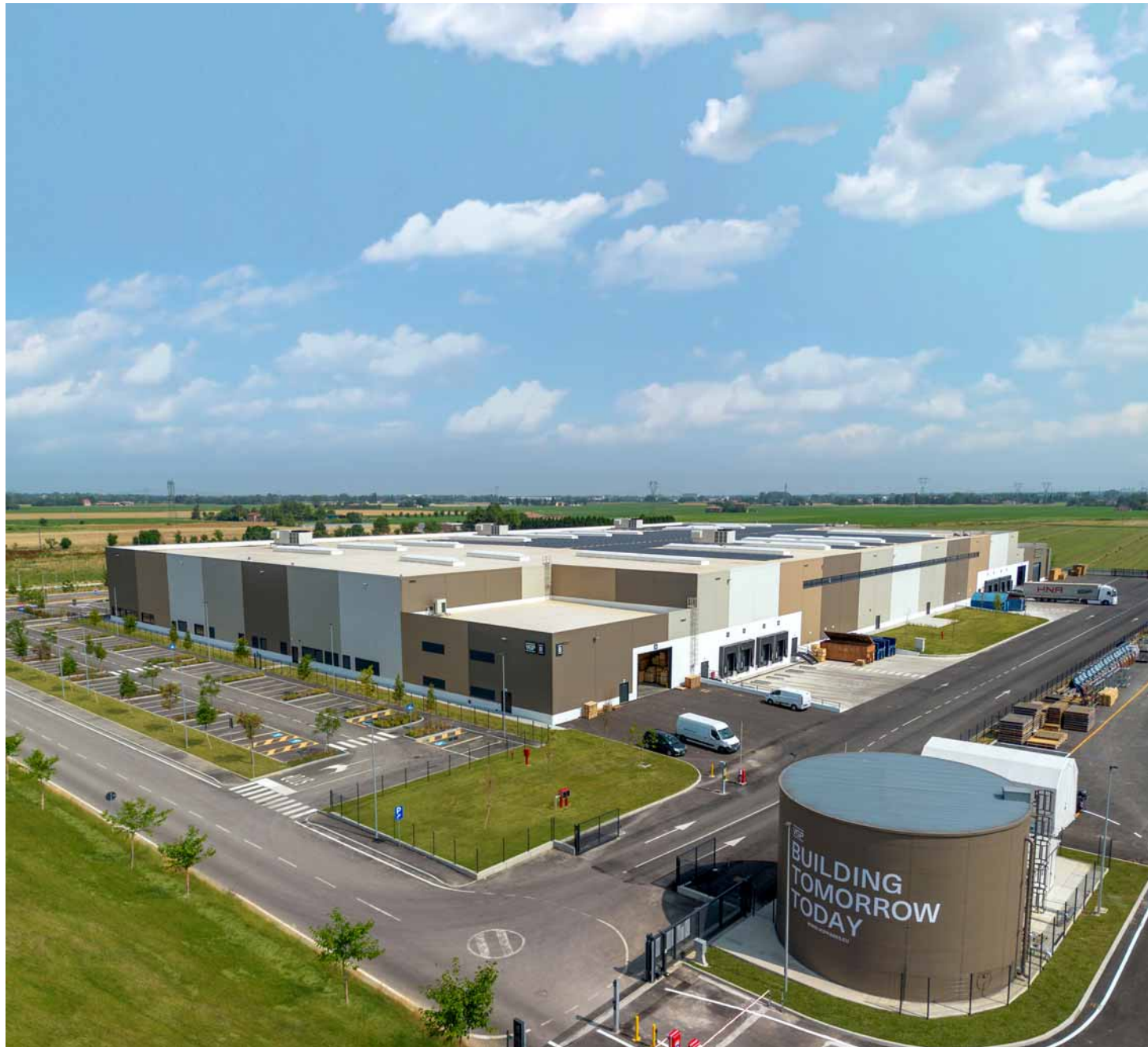
VGP Park Valsamoggia 2, Italy
