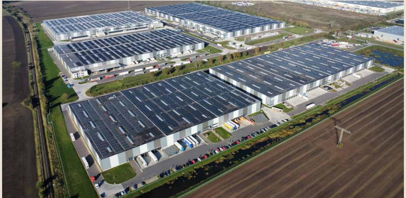
VGP Park Magdeburg is home to one of Germany's largest roof-fitted solar systems, with a capacity of 10.27 MWp. This system is part of a larger initiative where the entire VGP Park Magdeburg site has a total installed capacity of 25+ MWp
