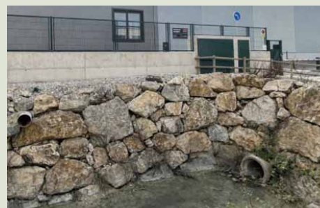
Dry-stone habitat structures integrated with the park's drainage system create small ecological niches for wildlife while supporting sustainable water management
