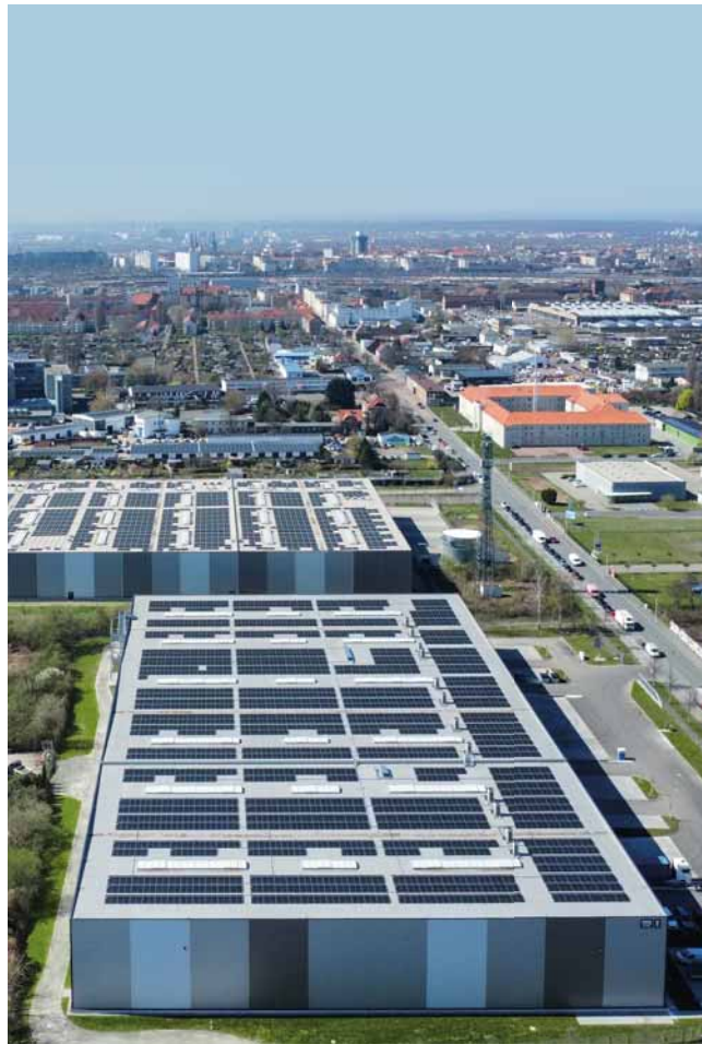
VGP Park Halle 2, Germany
