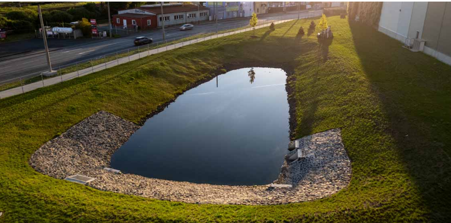
Climate adaptive water buffer at VGP Park Ústí nad Labem, Czech Republic
