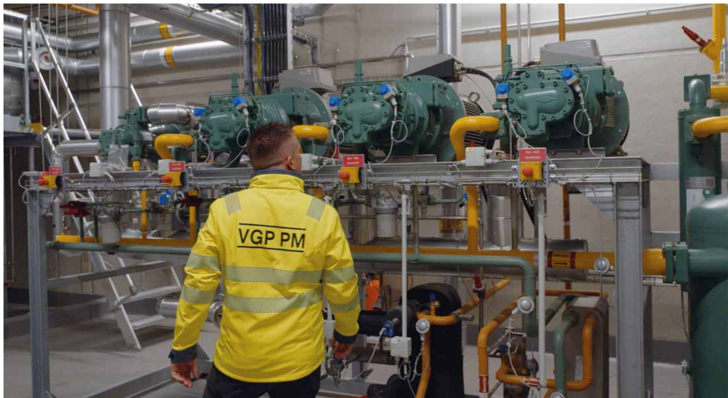
Maintenance in VGP Parks
