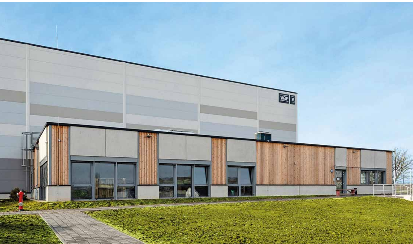
Partial wooden façade at VGP Park Hochheim, Germany
